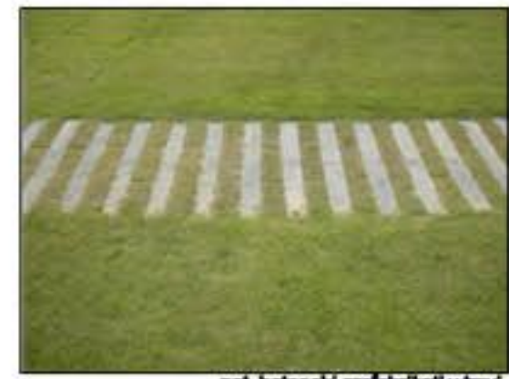
pot_betonaki prelazniki v travi
